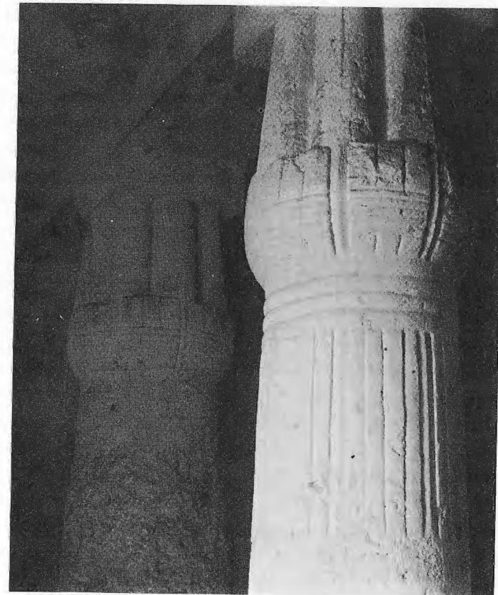
Plate 64. Capital of a bud column from a rock tomb at 'Amarna; the column to the rear was left unfinished.
